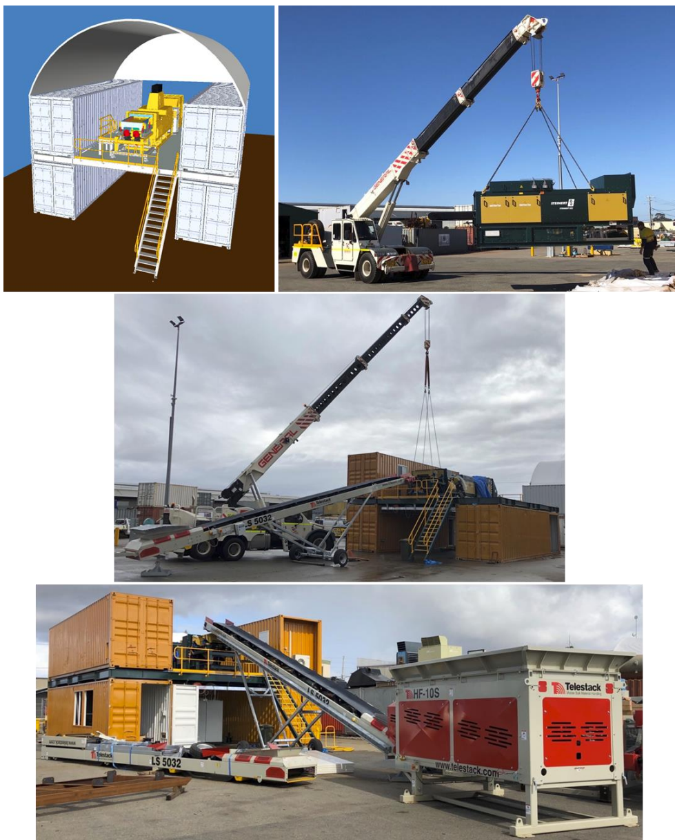
(Figure 2 - NavisWorks vs. Actual Sorter plant during construction.)
