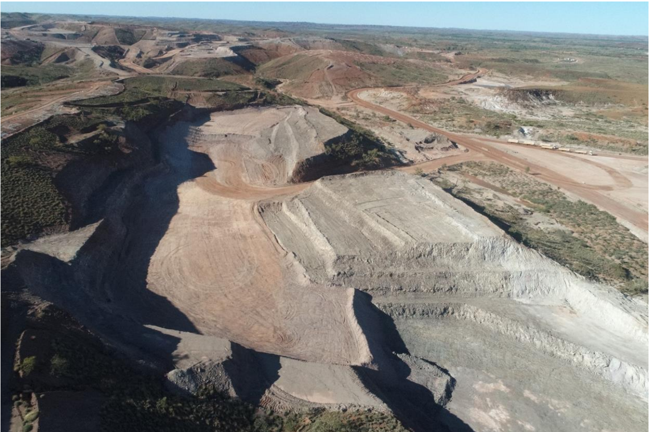
Figure 3: Grant's Hill pit with requisite backfilling complete.
